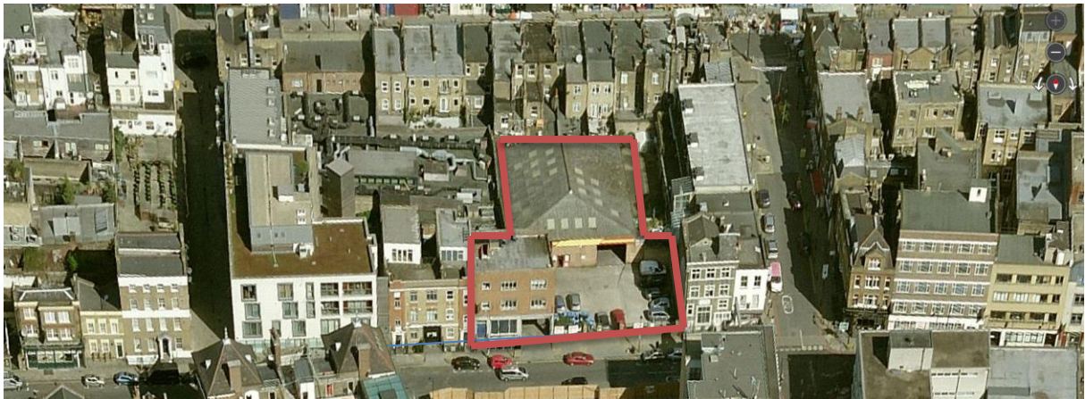
Aerial view of site from the south
